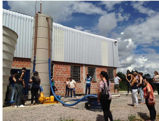
UASB reactor Application: Biogas production
